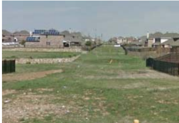
Spillway and draining area at Western side of property.
