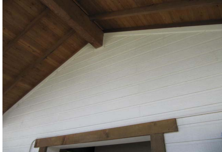
Composite siding at pool house exterior.
