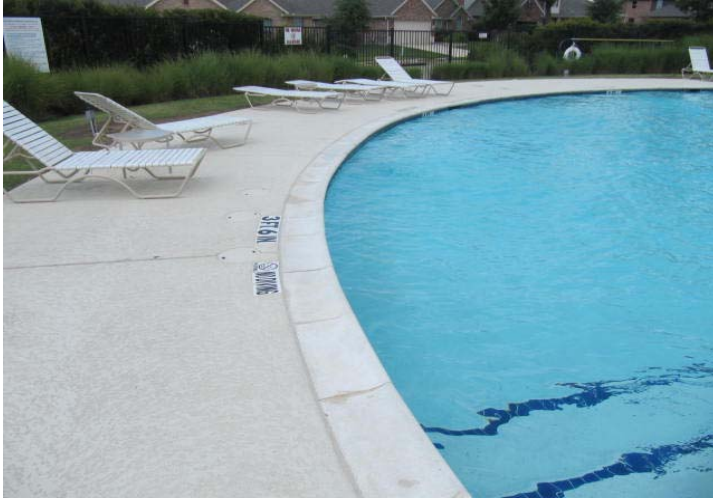
Pool coping at perimeter of swimming pool.
