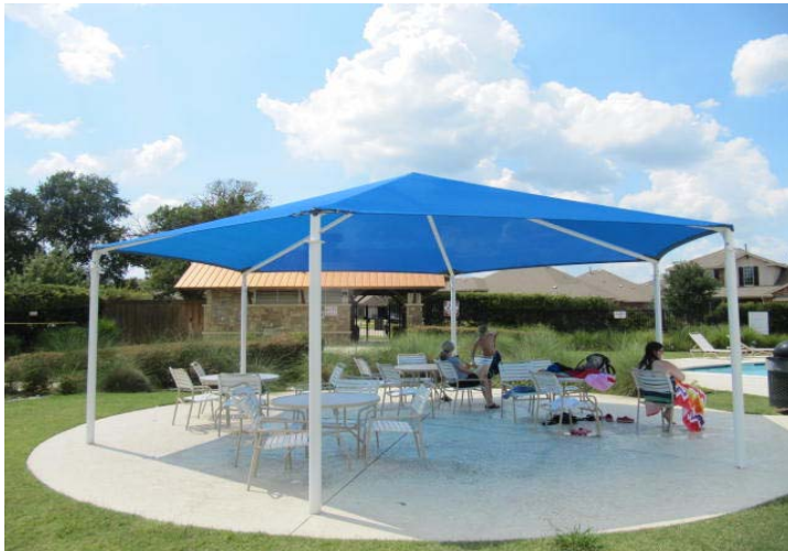
Overview of sunshade structure.
