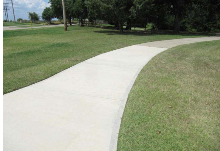
Newer section of concrete flatwork.
