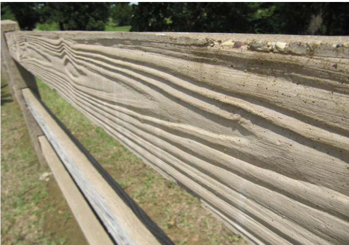
Typical textured formed concrete fence rail.
