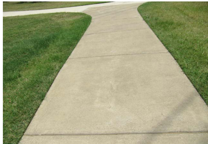
Concrete sidewalk at walking trail.
