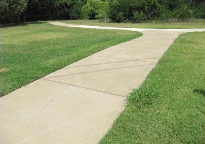
Overview of concrete sidewalks at walking trail.
