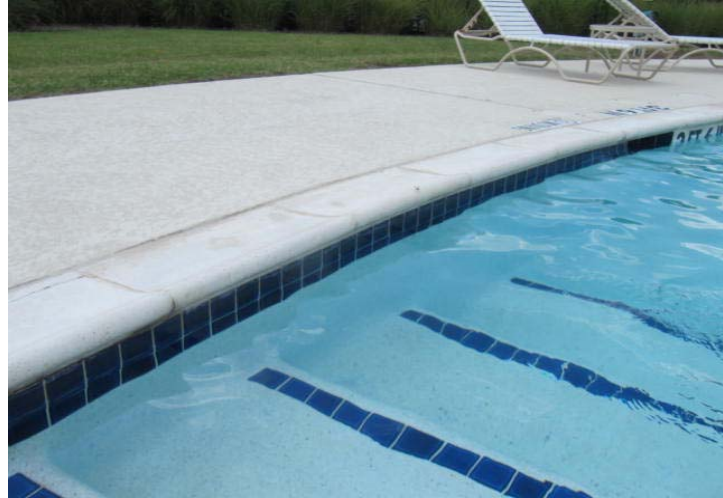
Pool coping at perimeter of swimming pool.
