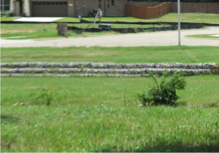
Gabion wall at common area.
