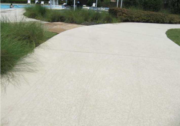
Overview of textured pool deck.
