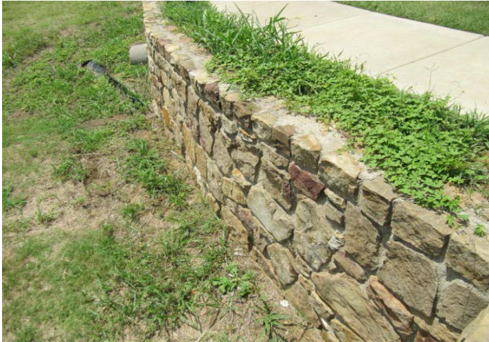
Retaining wall at end of cul-de-sac.
