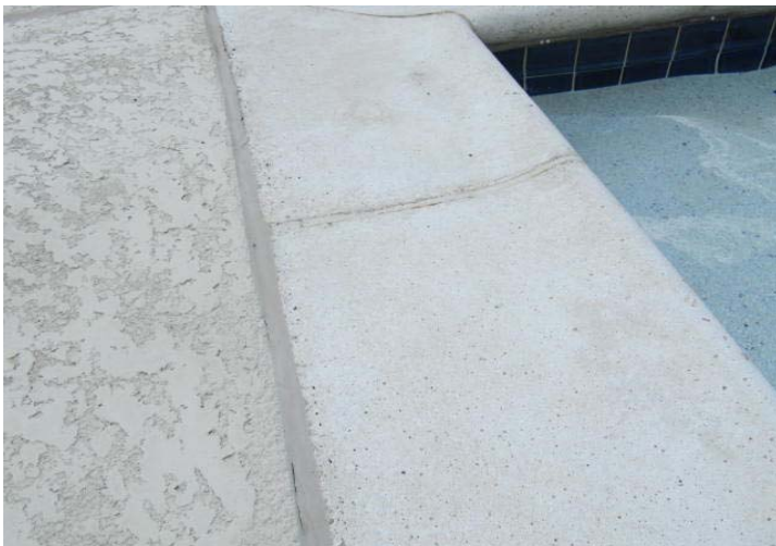
Formed concrete coping at perimeter of pool.
