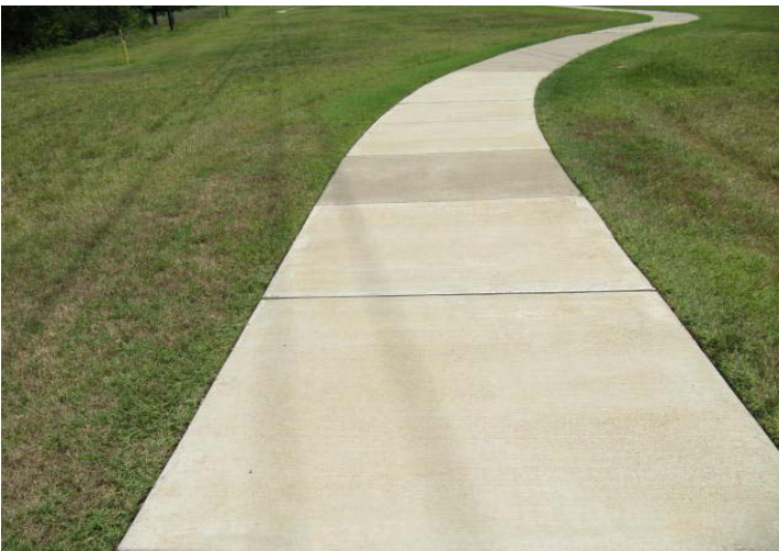
Concrete flatwork, of varying ages.
