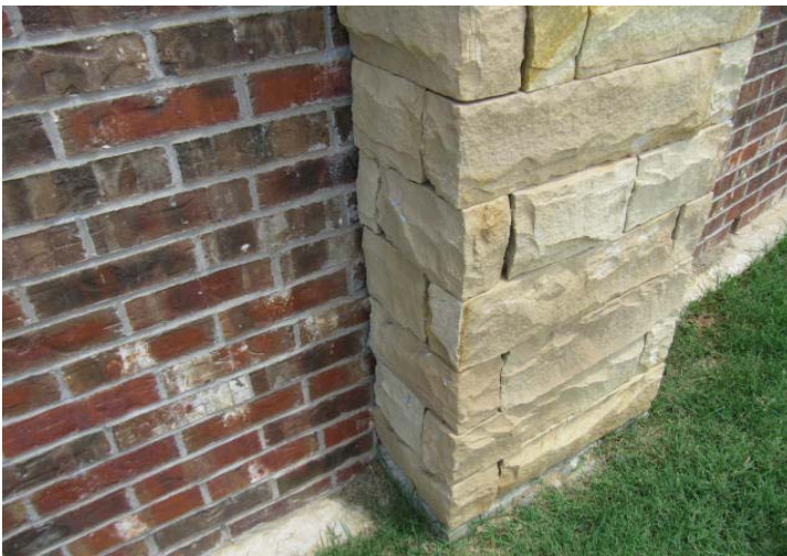
Brick wall panel and stone pier at property perimeter.
