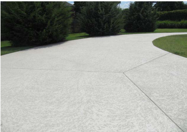
Pool deck in good condition, with no cracks.
