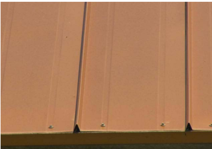
Aluminum standing seam roof at pool house.
