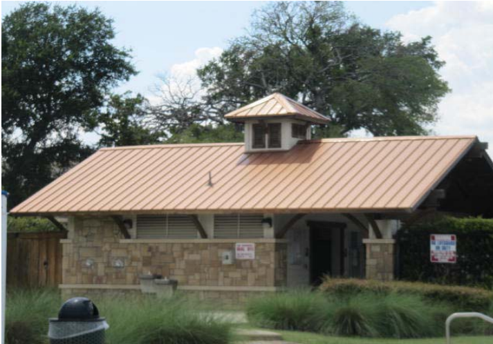
Overview of exterior of pool house.
