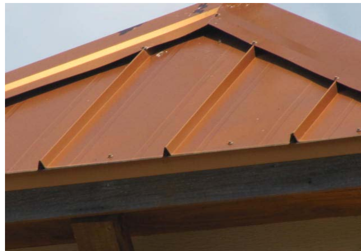
Good finishes at metal roof panels.
