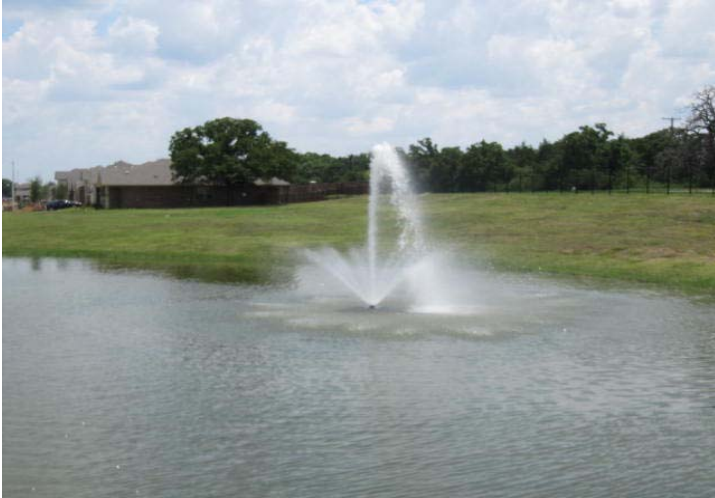
Overview of pond aerator.
