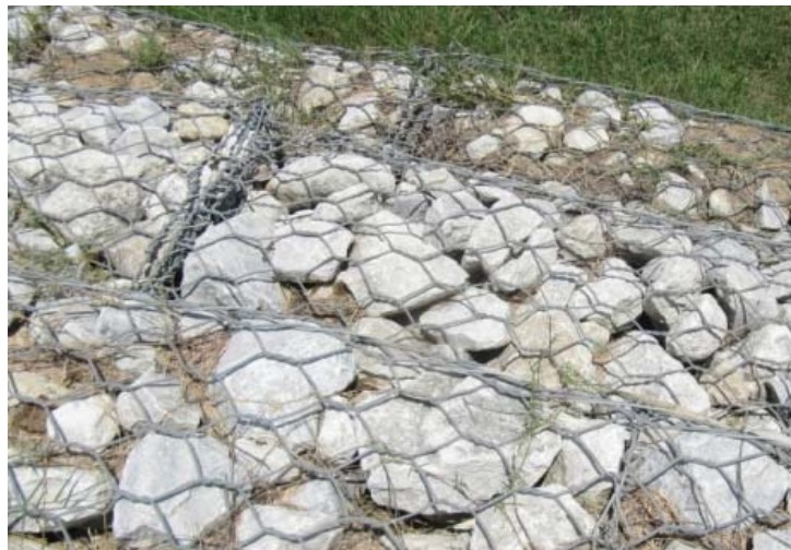
Terraced steps at gabion wall.
