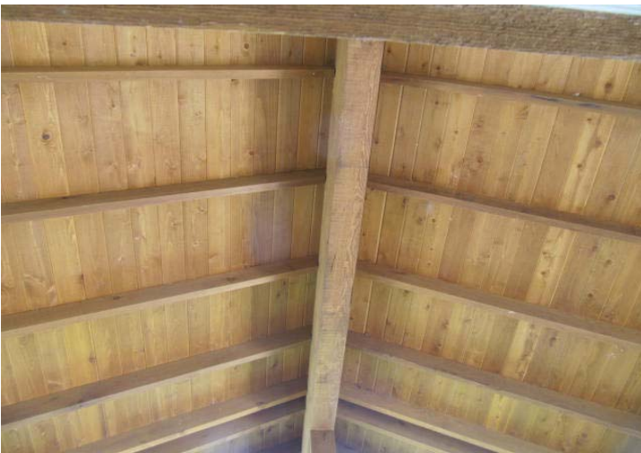
Tongue and groove ceiling at pool house.
