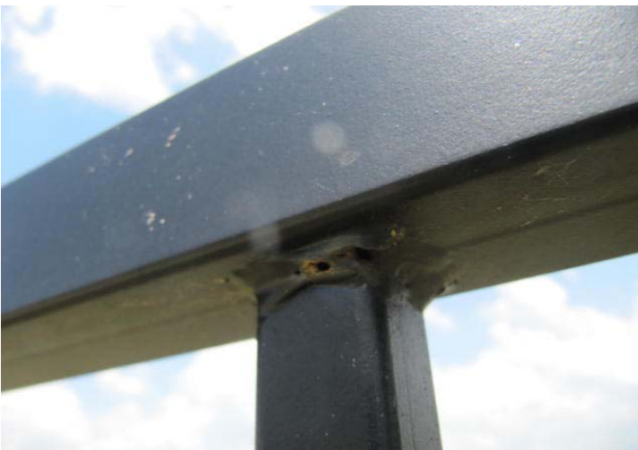
Typical condition of finishes at metal fence.
