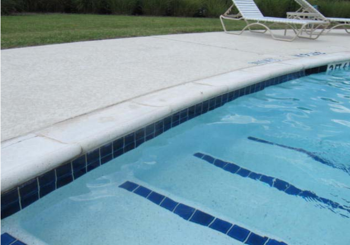
Overview of waterline tile at swimming pool.
