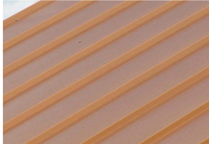
Aluminum standing seam roof at pool house.
