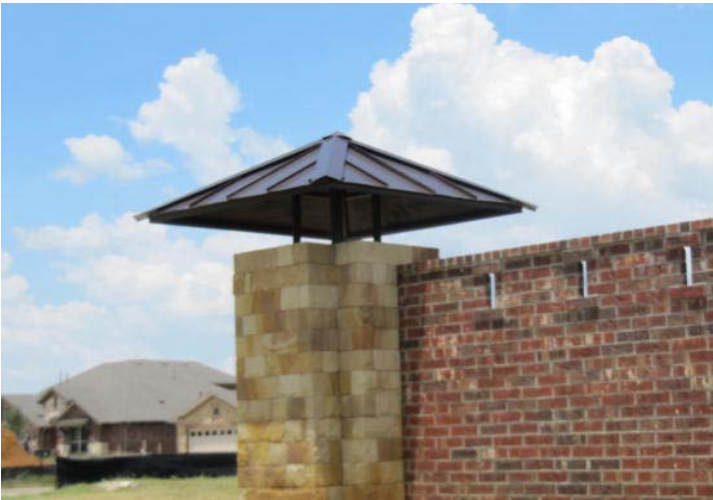
Overview of metal roof structure at perimeter wall.
