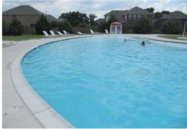
Diamond-Brite finish at pool interior.
