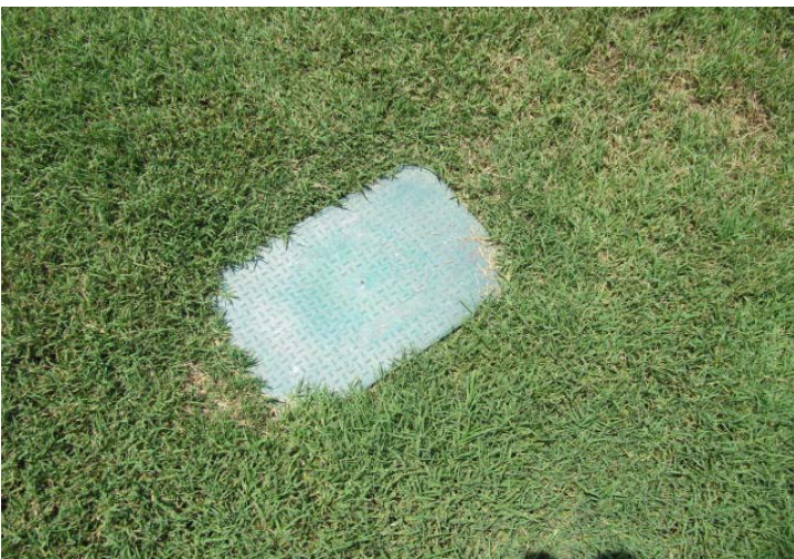
Cover at irrigation control valve.
