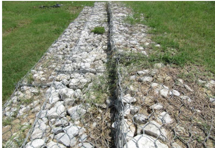
Stones and wire enclosure at gabion wall.
