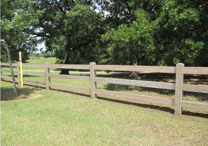
Overview of rail style fence.
