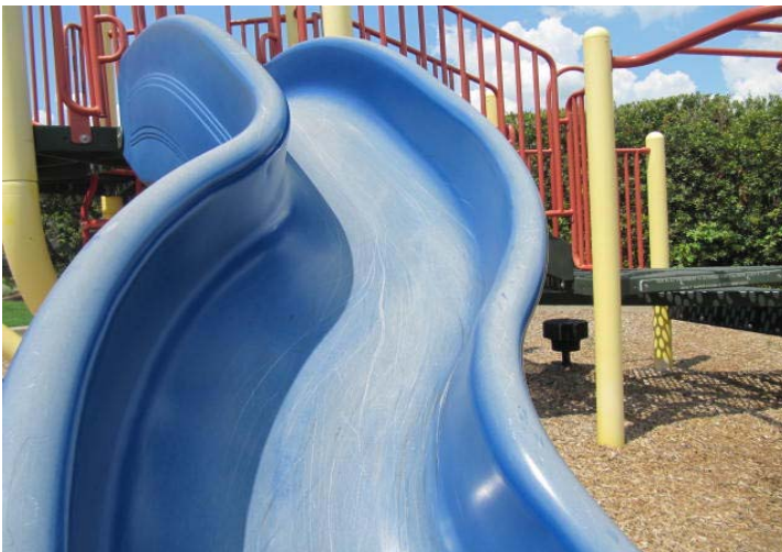
Markings at playground slide.
