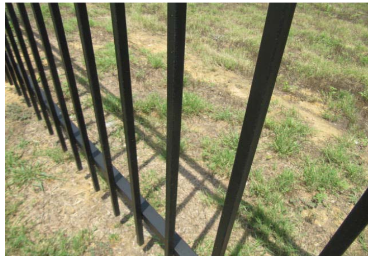
Typical metal pickets at fence.
