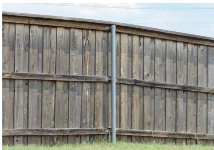
Typical metal post at rear of fence, with wood pickets.
