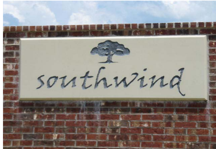
Precast signage at perimeter wall.
