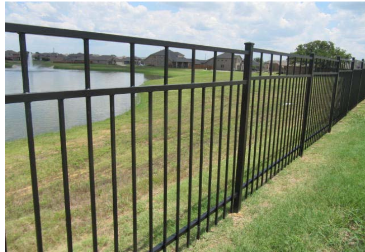
Overview of metal fence at property perimeter.
