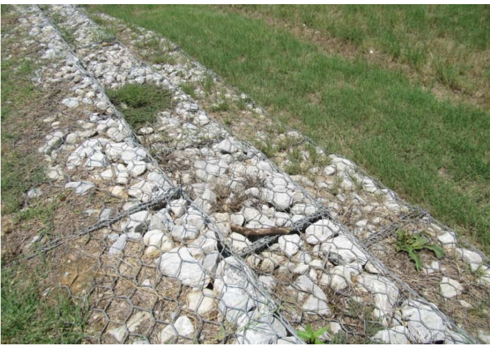
Stones and wire enclosure at gabion wall.
