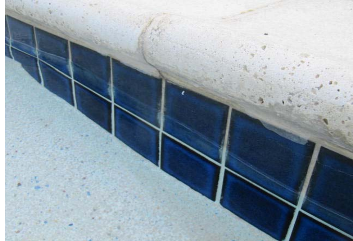
Typical condition of waterline tile at pool perimeter.
