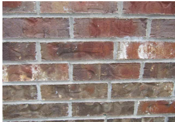
Typical condition of bricks and mortar joints.
