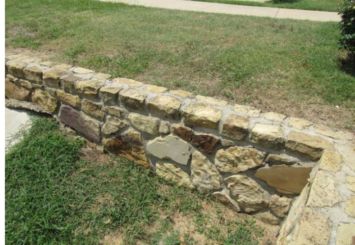
Retaining wall at end of cul-de-sac.
