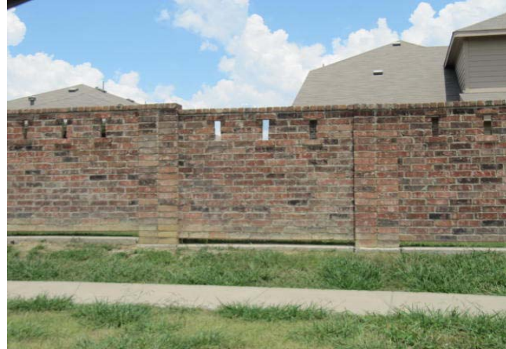
Overview of masonry perimeter wall.
