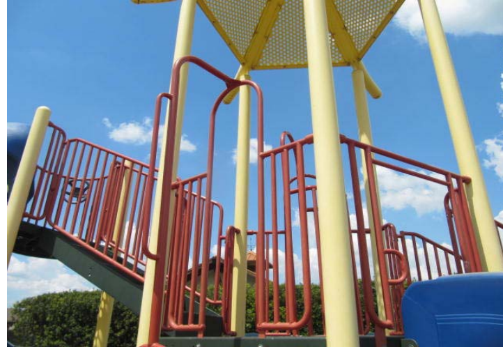
Tower and rails at playground structure.
