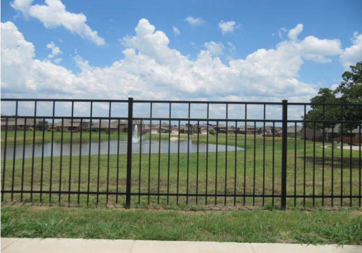
Overview of metal fence at property perimeter.
