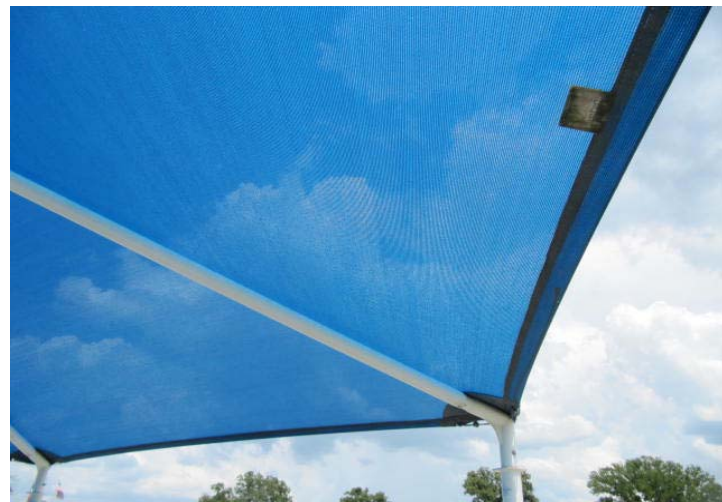
Original sunshade, in good overall condition.
