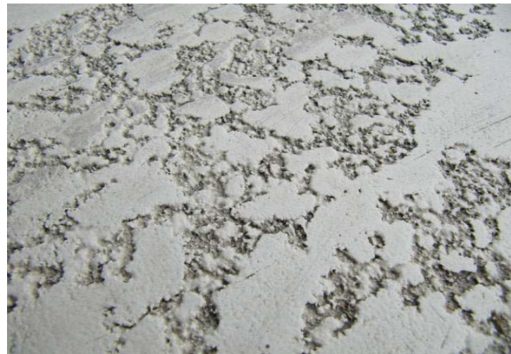
Typical texture at pool deck.
