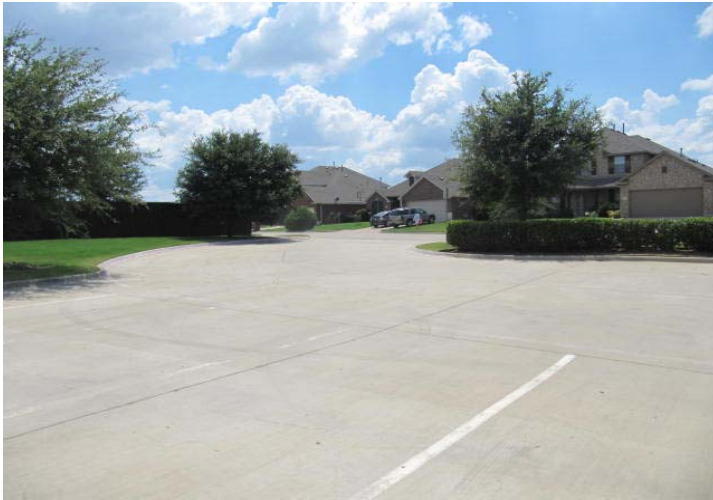
Overview of concrete parking lot.
