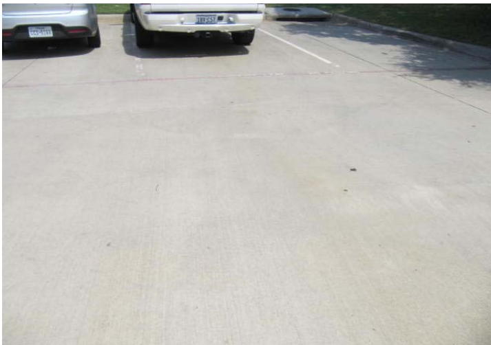
Typical condition of concrete flatwork at parking lot.
