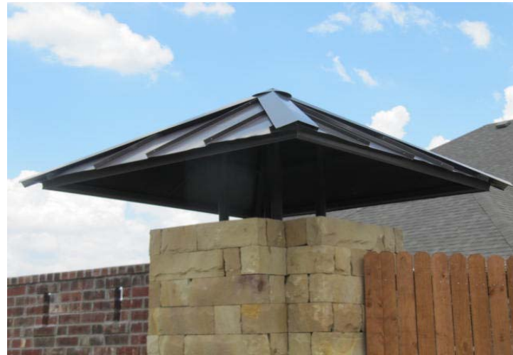
Peaked roof at monument signage, at property perimeter.
