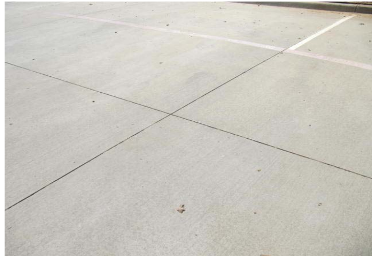
Concrete flatwork, with saw-cut control joints.
