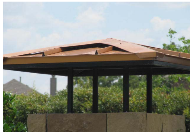
Roof structure at monument near swimming pool.
