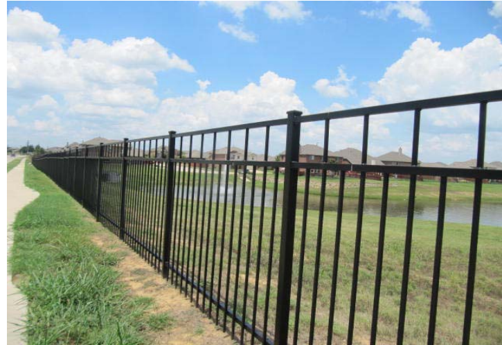
Metal picket style fence, in good condition.
