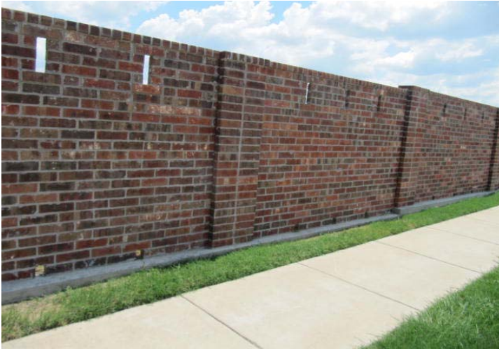
Overview of masonry perimeter wall.
