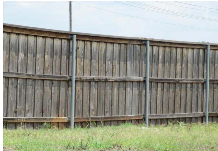
Wood privacy fence along transmission line easement.
