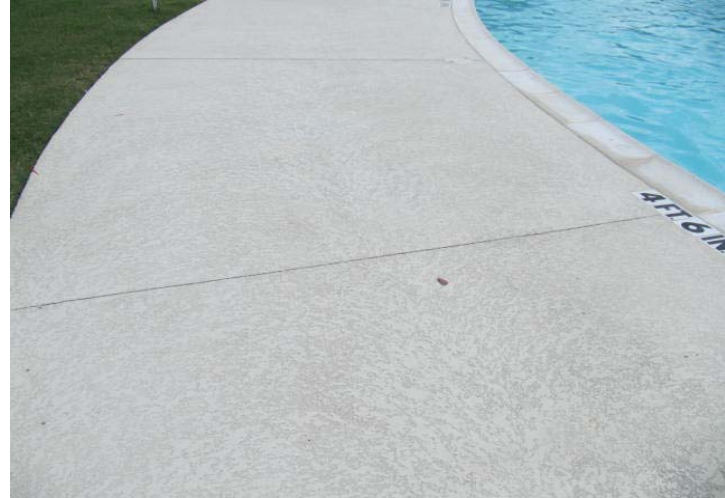
Spray deck surfacing at concrete pool deck.
