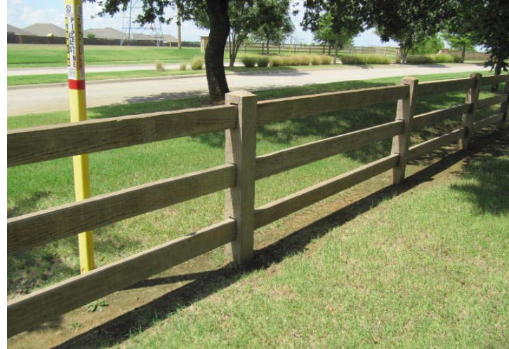
Concrete 3-rail fence, in good condition.
