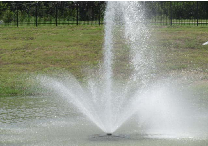
Pond aerator, in good functional condition.
