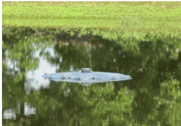
Non-operational aerator at front pond (low water level).
