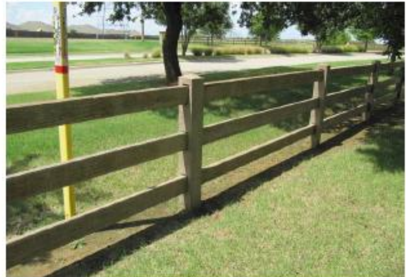
Concrete 3-rail fence, in good condition.
